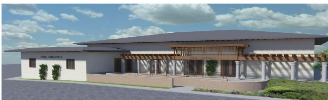
Parish Hall Expansion, looking South from the Parish Office
